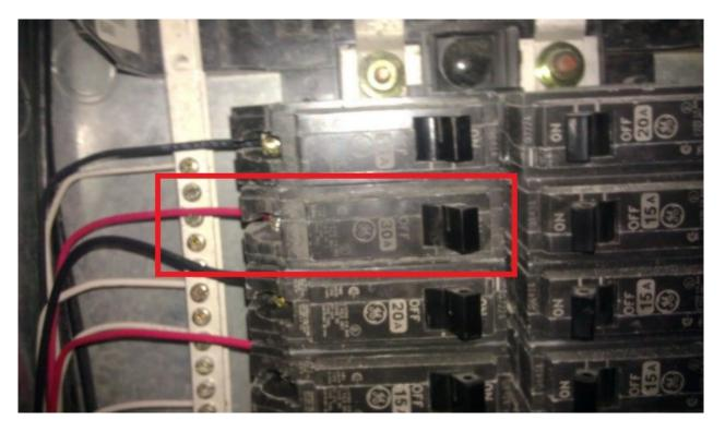
Unsafe connection is noted in the main electrical panel (30AMP breaker connected to a 14 AWG wire).
