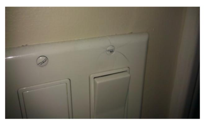
The light switch cover plate in the bedroom is unsafe (cracked) and it should be replaced.
